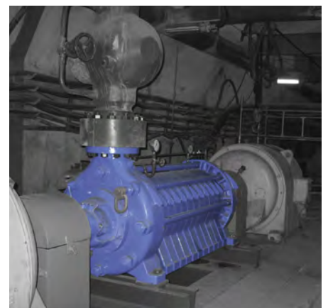
Intermediate flange at stage casing
